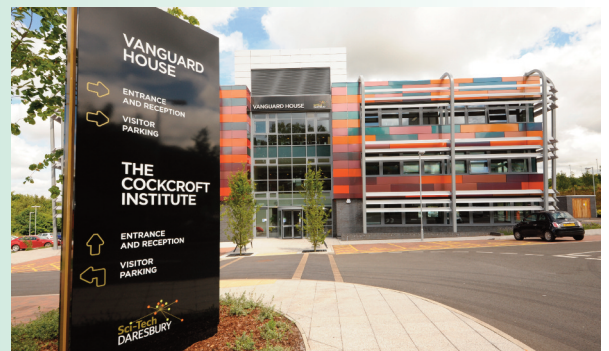
Vanguard House opened in June 2011 to accommodate the growing businesses at Sci-Tech Daresbury.
